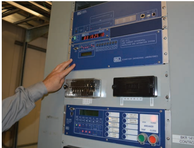
Relay panels inside the control building tell circuit breakers when to open and close.
