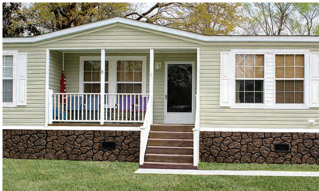
To save money on your energy bill, add skirting around your manufactured home. PHOTO COURTESY OF WINFIELD SUPPLY
